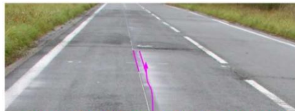
300 m of road equipped with a neutral coloured magnetic tape
